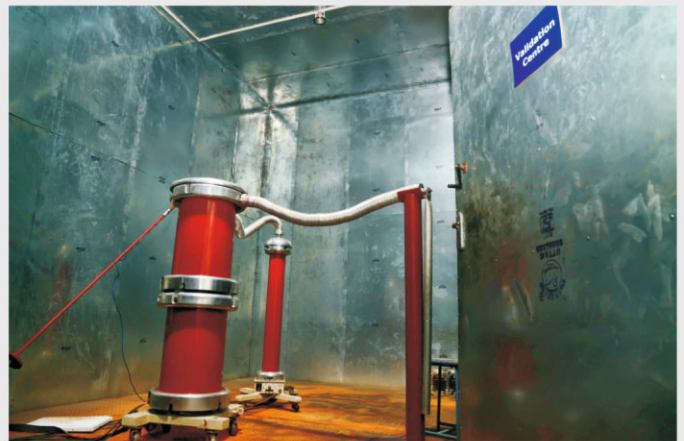
Partial Discharge Test
